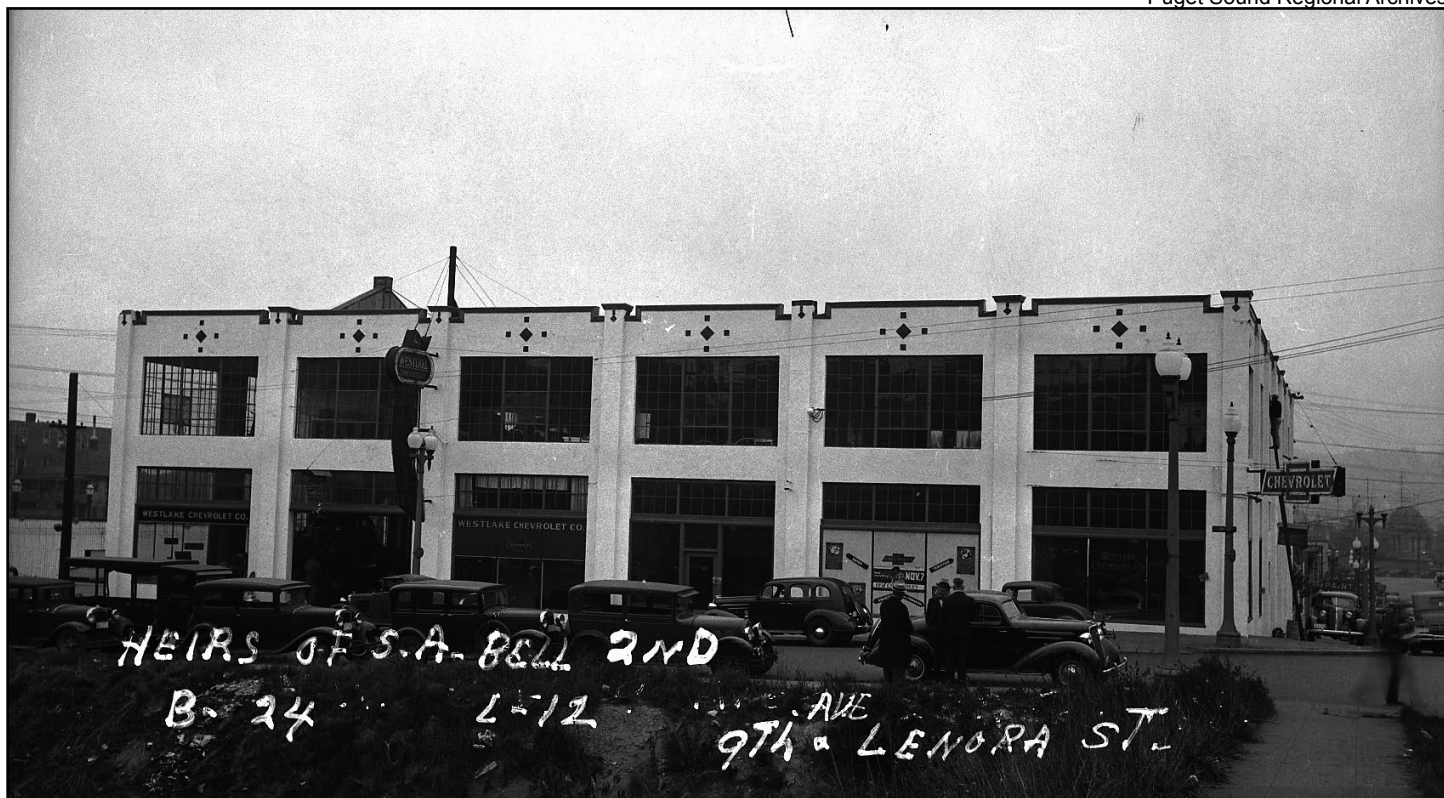
Figure 44 • Garage Building for George L. Seibert, Westlake (Earl Roberts, 1924)
