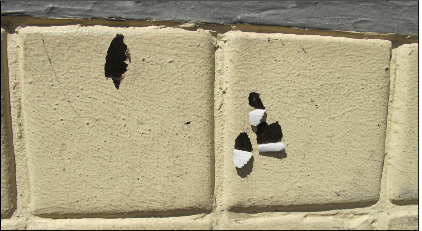
Figure 12 • Eldridge Tire/1519 Broadway, detail of tile
