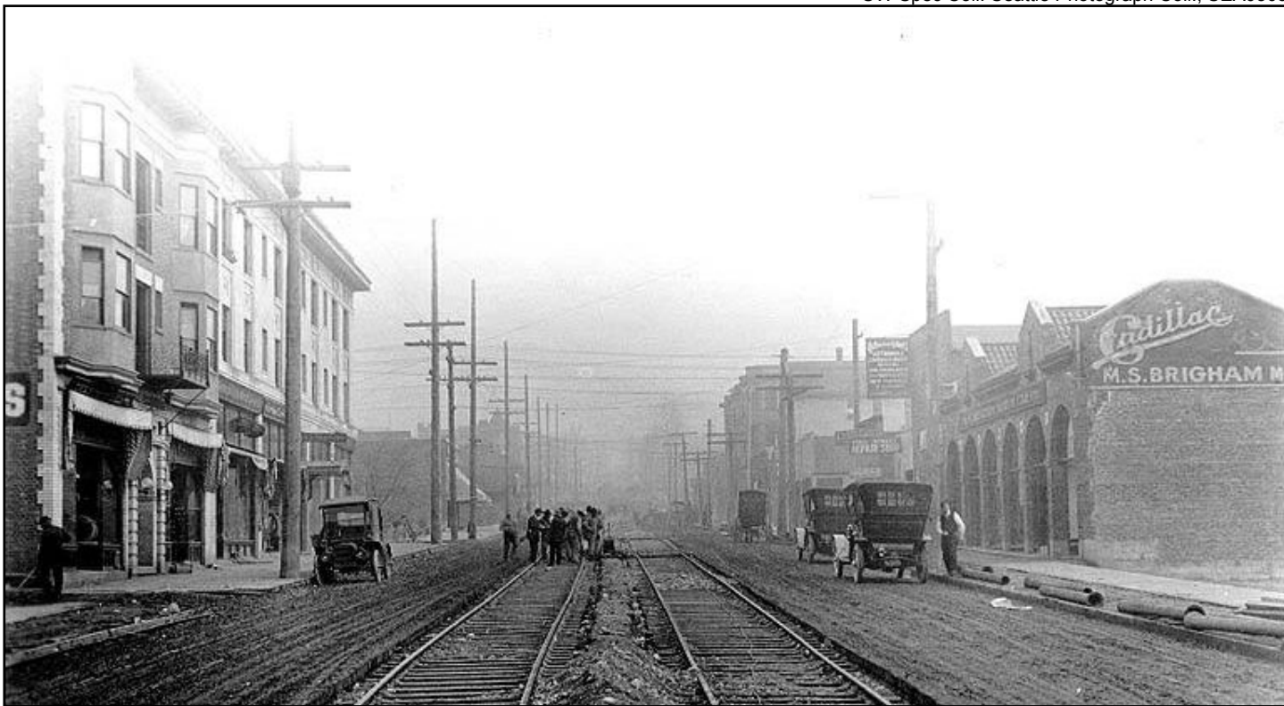
Figure 18 • Pike Street from Broadway Avenue E, 1911
