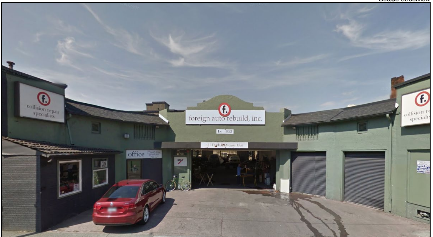
Figure 38 • Garage for A. A. Bain and A. D. Schafer/Pontius Garage, 421 Eastlake Avenue (William Bain, Sr., 1926)
