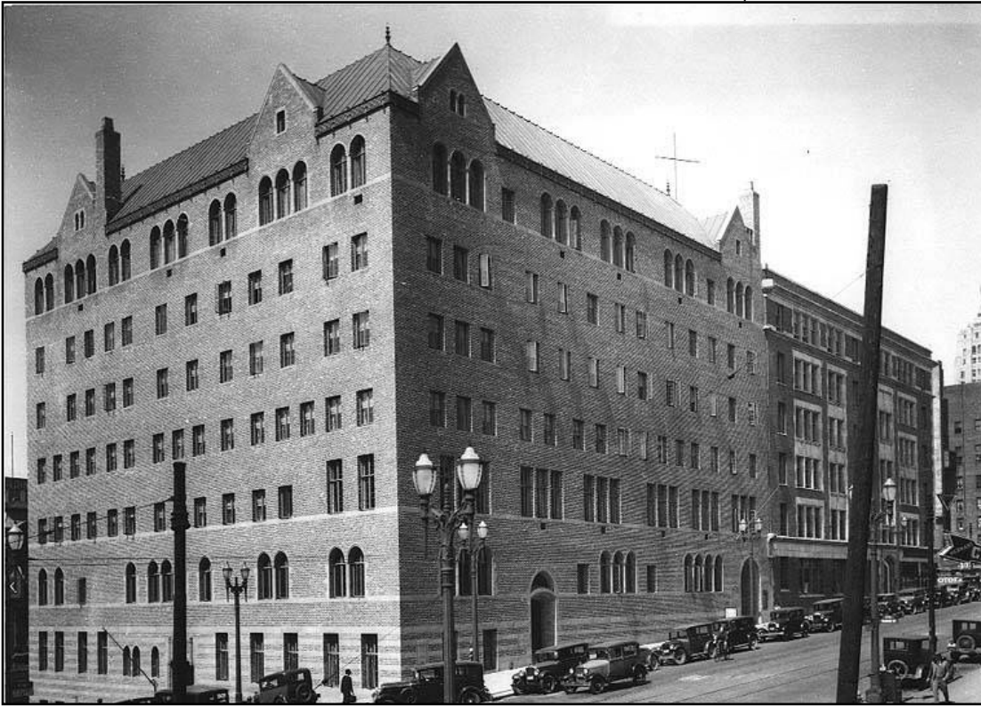
Figure 57 • Downtown YMCA (A. H. Albertson & Associates, 1929-31, City of Seattle Landmark)
