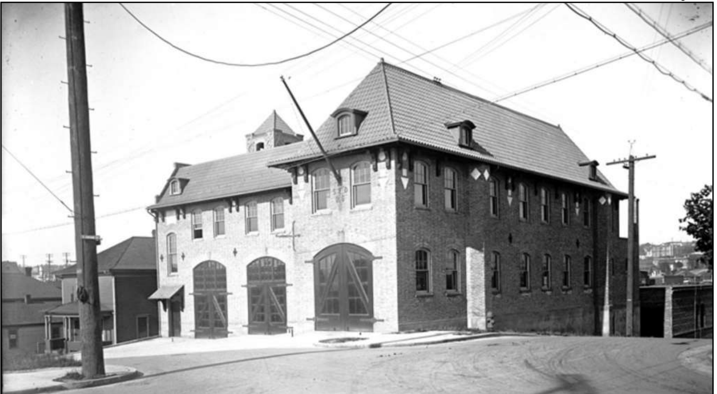
Figure 26 • Old Fire Station #25, 1400 Harvard Avenue (Somervell & Cote, 1909, City of Seattle Landmark)
