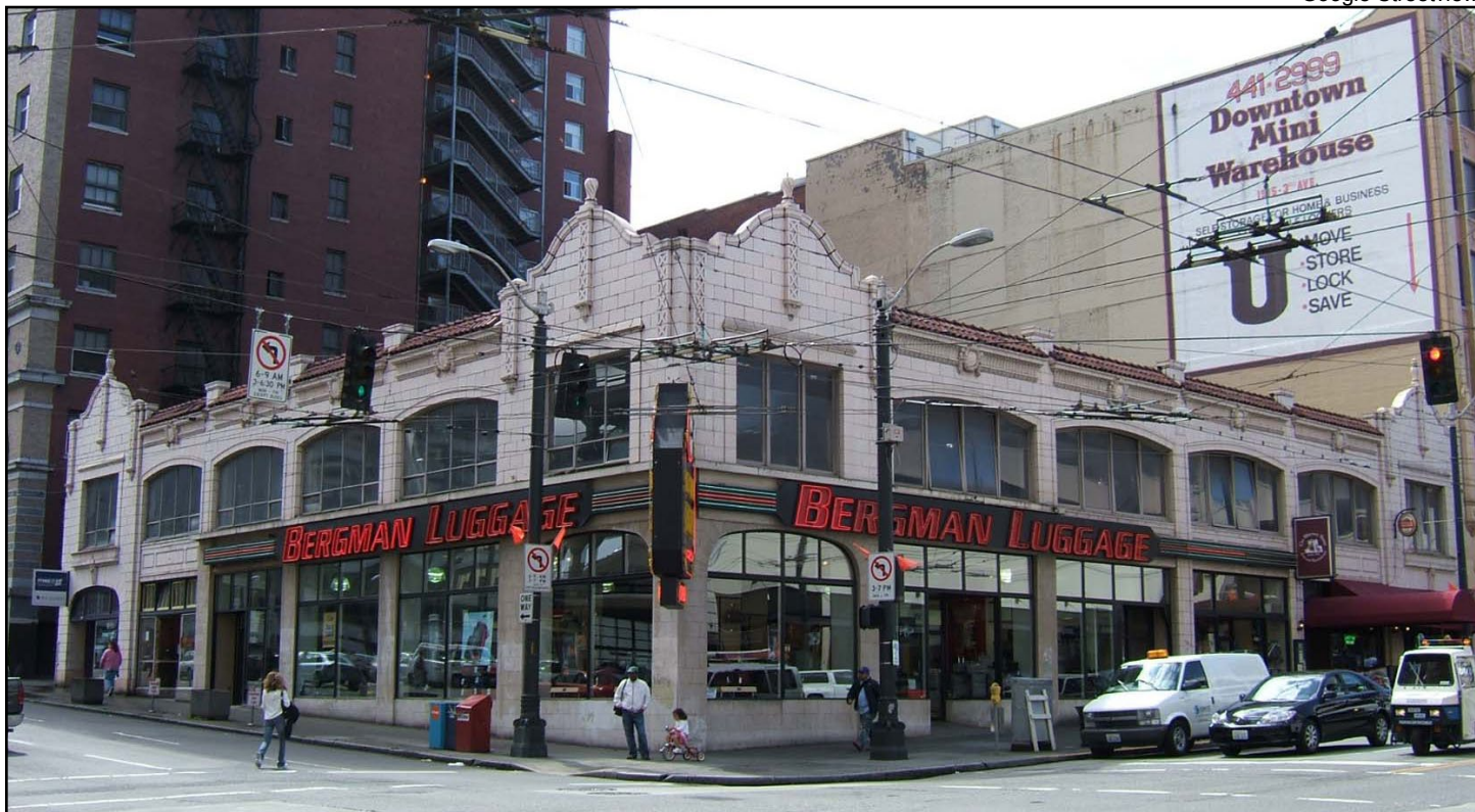
Figure 45 • Former Donahoe Garage (Charles Haynes, 1916)
