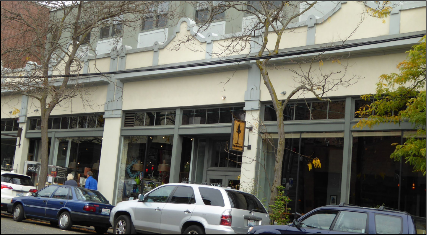
Figure 39 • Wilson Motor Company, Ballard Avenue (1905, 1923)
