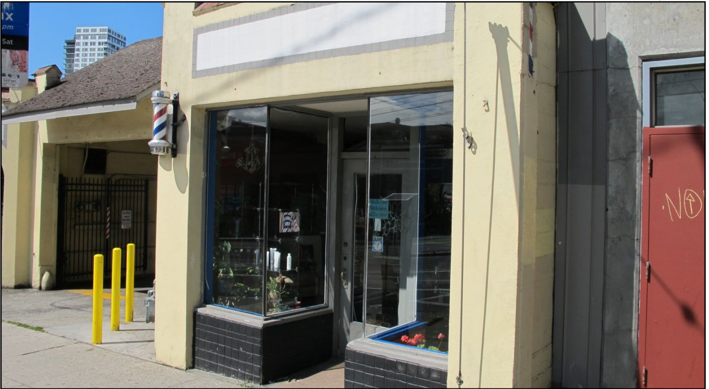
Figure 7 • Eldridge Tire/1519 Broadway, northern storefront
