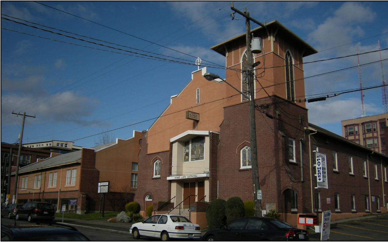
Figure 29 • First African Methodist Episcopal Church, 1522 14th Avenue (1912, City of Seattle Landmark)
