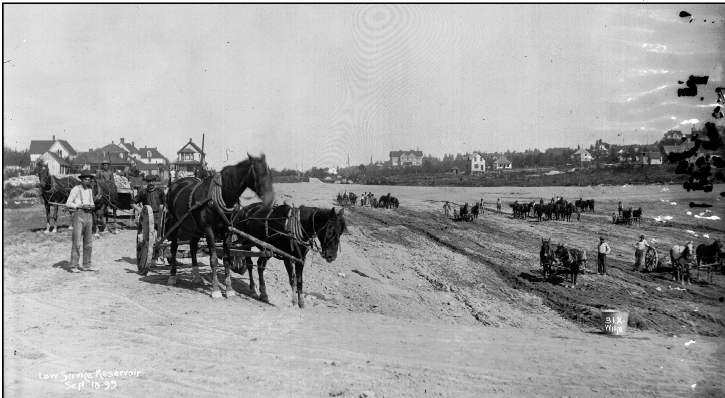
Figure 17 • Lincoln Reservoir under construction, September 18, 1899
