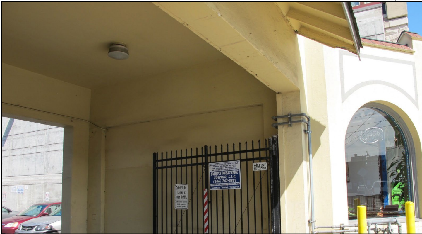
Figure 10 • Eldridge Tire/1519 Broadway, northern storefront & porte-cochère
