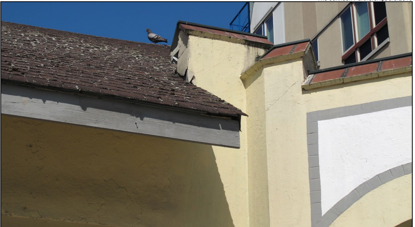
Figure 9 • Eldridge Tire/1519 Broadway, detail at roof
