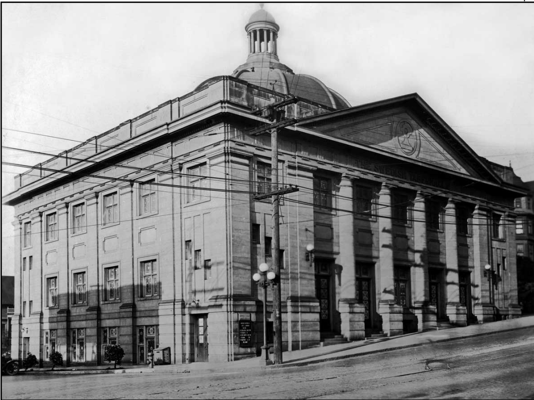
Figure 24 • First Covenant Church, 1500 Bellevue Avenue E (John Creutzer, 1910-1911, City of Seattle Landmark)
