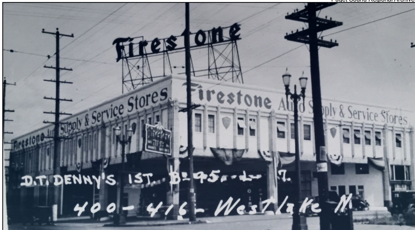
Figure 46 • Firestone Tire, 400 Westlake Avenue (The Austin Company, 1930, City of Seattle Landmark)
