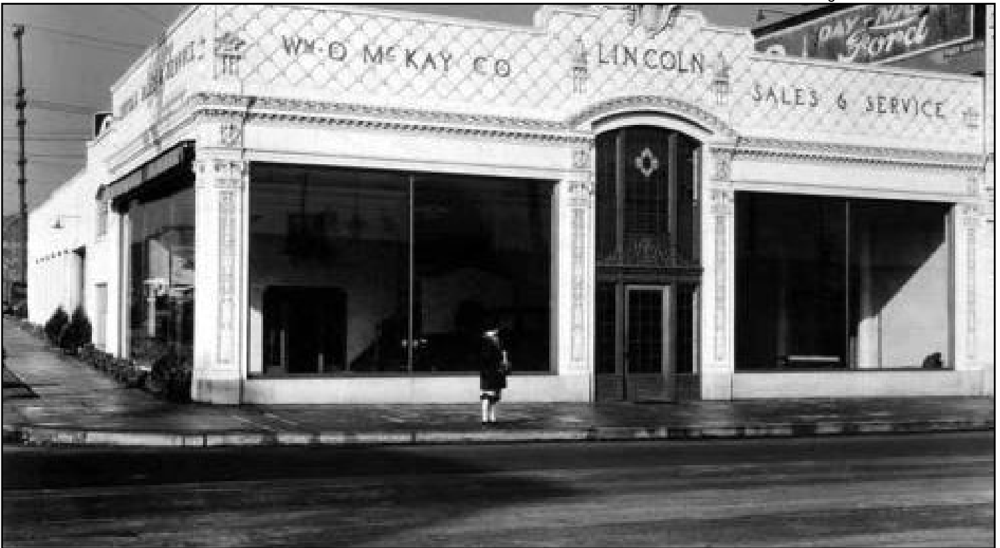
Figure 41 • The Pacific McKay Building (Harlan Thomas and Clyde Granger, 1925, City of Seattle Landmark)
