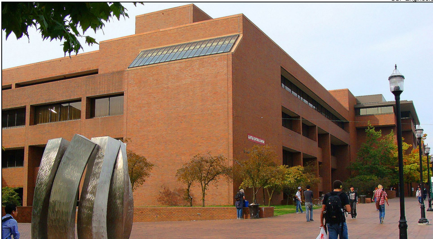
Figure 53 • Broadway Edison Building, Seattle Central College 2010 (NBBJ, 1979)
