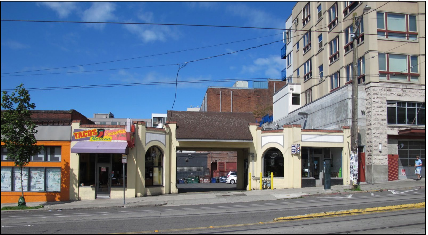
Figure 6 • Eldridge Tire/1519 Broadway eastern façade
